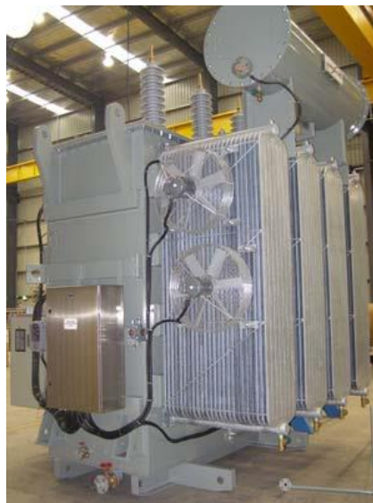
Oil Forced Air Forced or OFAF Cooling of Transformer
