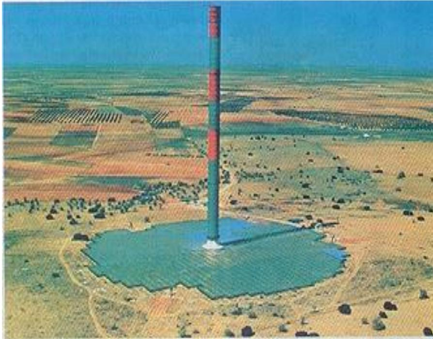
Pilot plant: only one big solar chimney has ever been built, the 195-metre prototype at Manzanares in Spain
